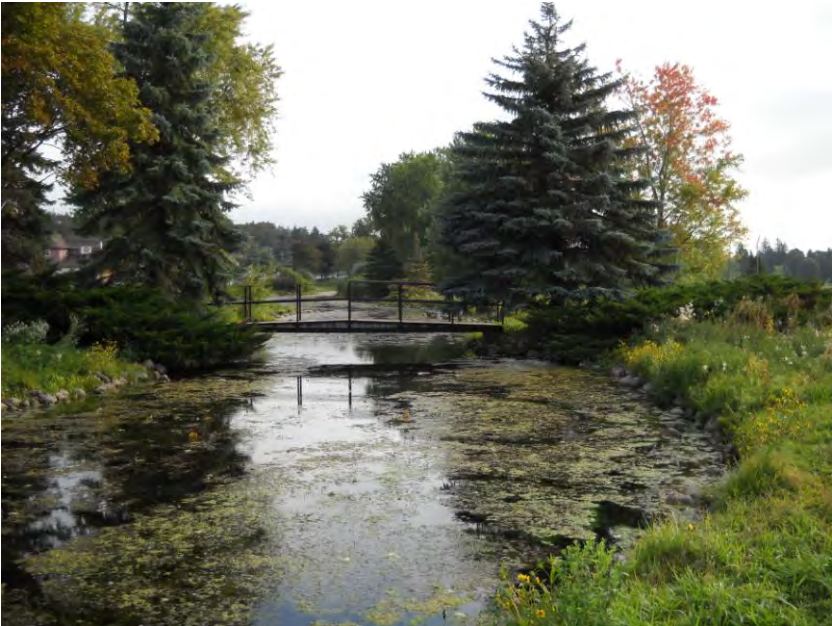
Pedestrian bridge over Clythe Creek
