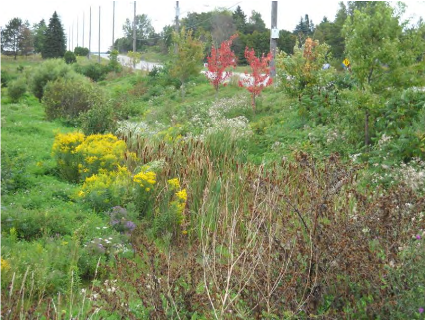
Victoria Road and Stone Road SWM Facility No. 104
