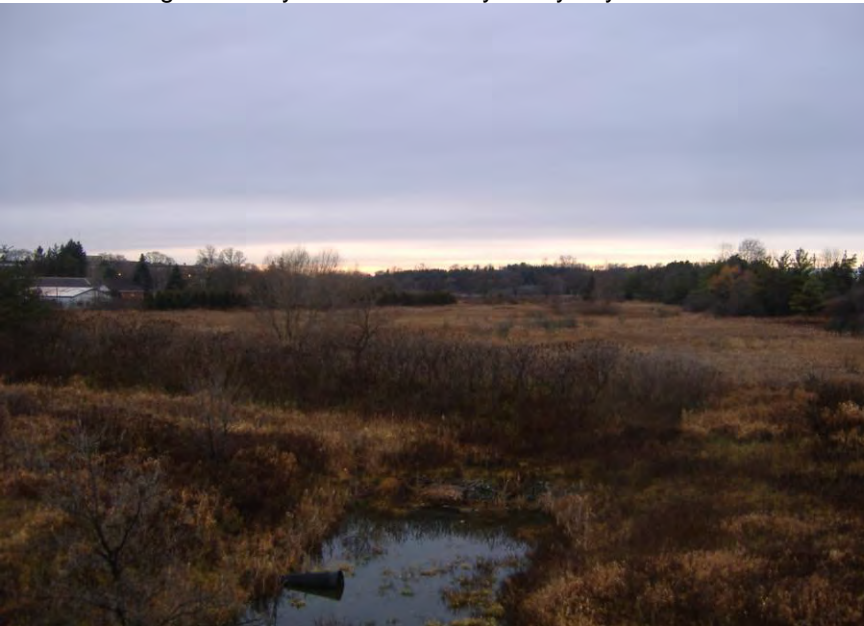
Channel around SWM Facility No 38
