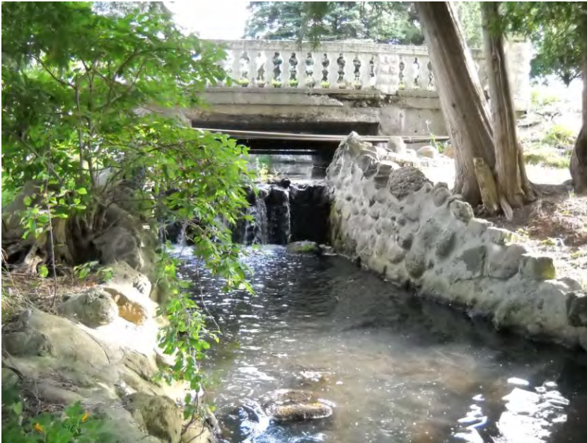
Correctional Facility bridge over connection between east & west ponds
