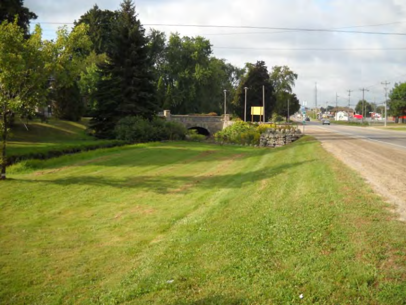
Clythe Creek next to York Road
