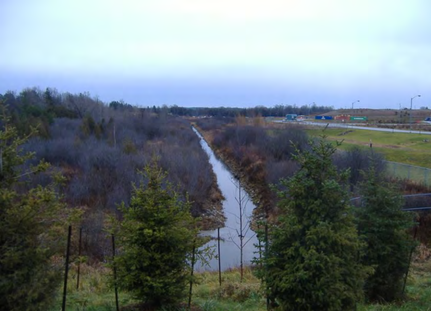
Channel adjacent to Watson Parkway south of Dunlop Drive
