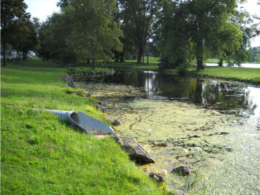
York Road drainage outlet to Clythe Creek
