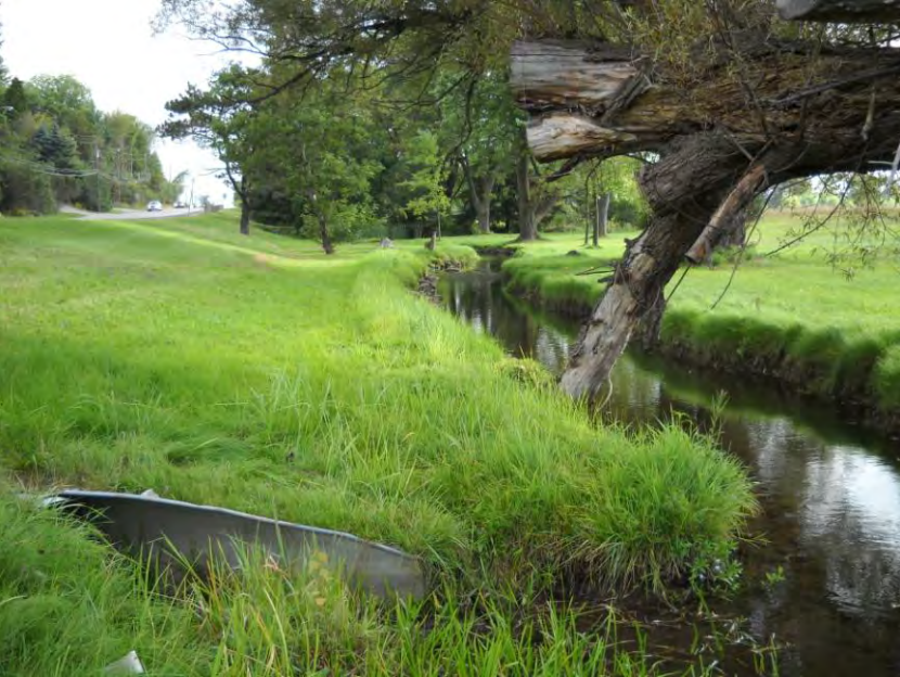
York Road drainage outlet to Clythe Creek
