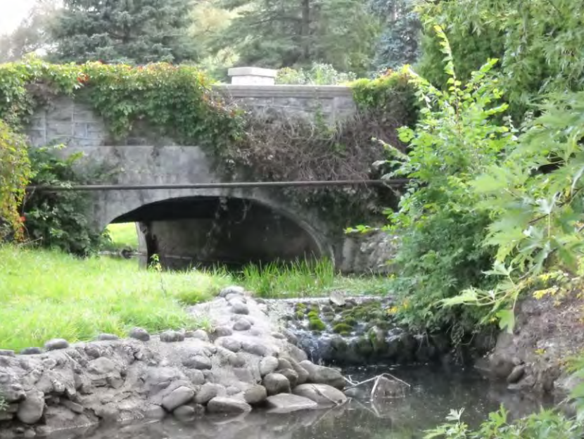
Drop structure and driveway to Correctional Facility
