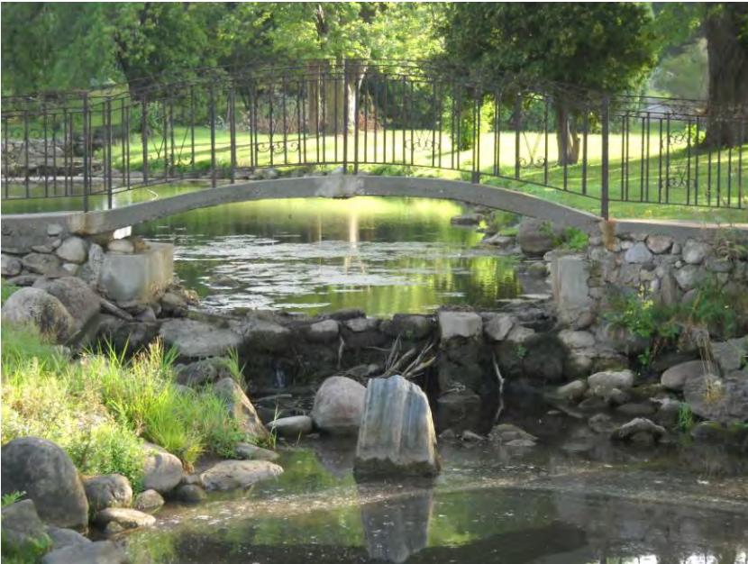
Pedestrian bridge and drop structure in Clythe Creek
