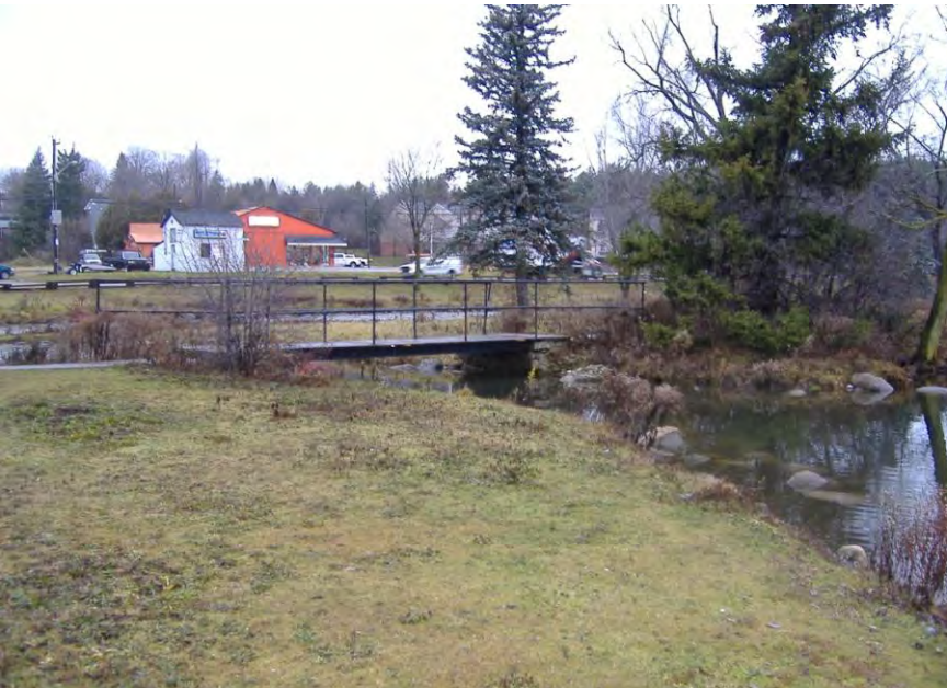
Bridge over Clythe Creek at Royal City Jaycees Park
