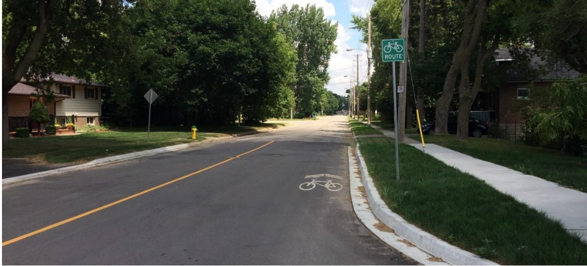
Figure 1 Signed routes are wayfinding strategies to direct cyclists through quiet residential areas connecting them to key commercial and employment hubs
