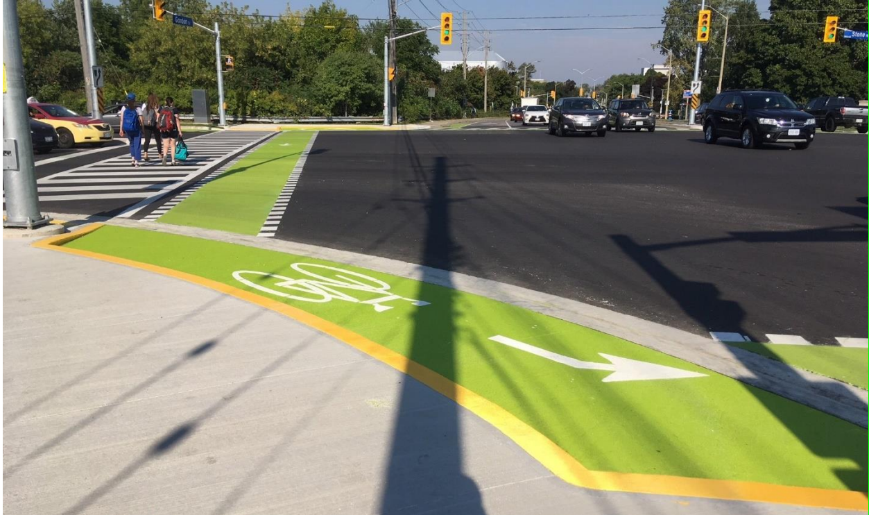
Figure 7 The new configuration at Gordon Street and Stone Road gives people who bike the option to turn left like a pedestrian does, instead of like a vehicle does.
