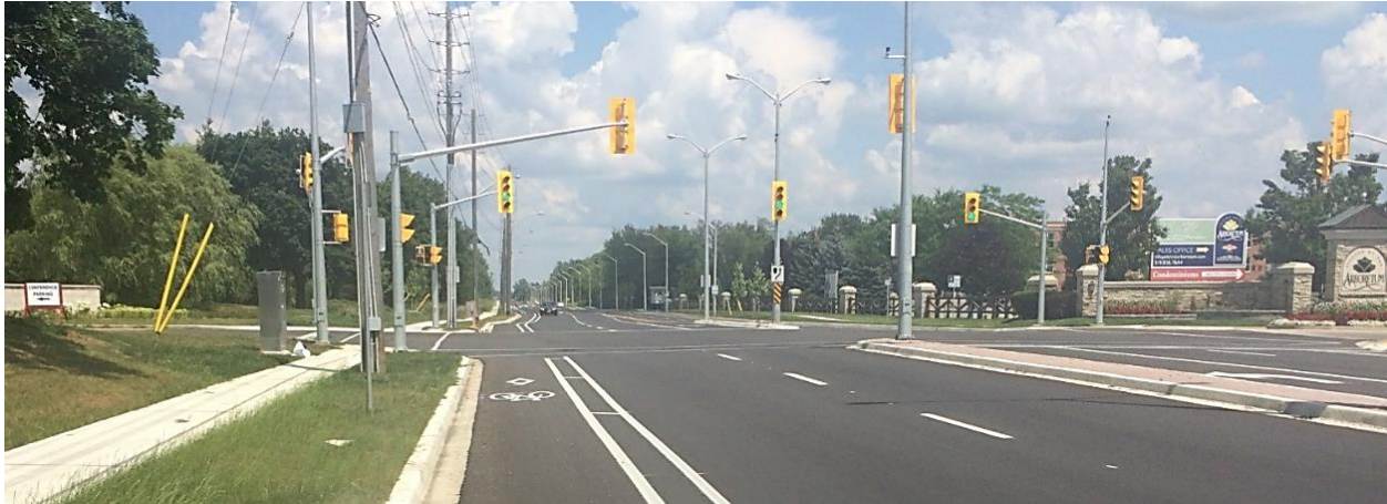
Figure 2 Bike lane on Stone Road in Guelph, featuring a painted buffer which creates additional space between bicycles and vehicles.
