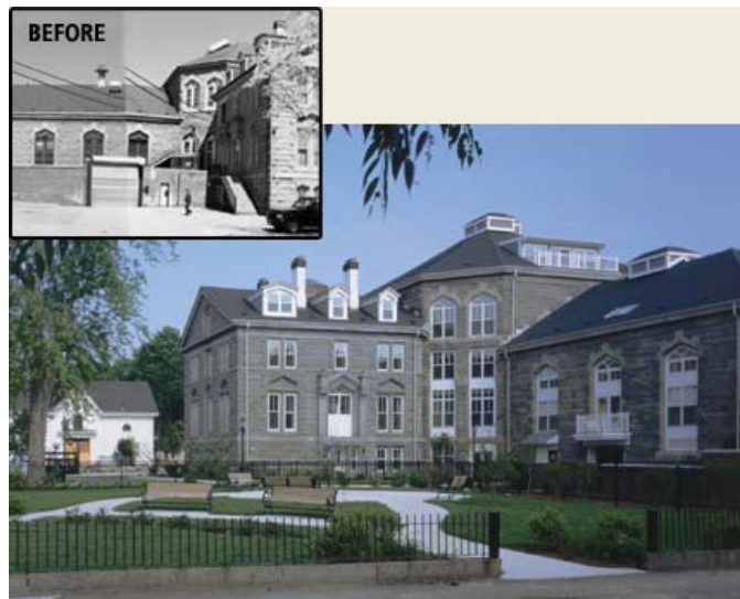
Figure 9 - Adaptive Reuse of Jails in Suffolk County, Virginia
