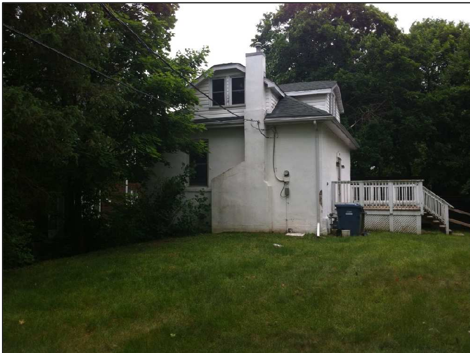
(Photos taken by R. Harris, June 2014)
